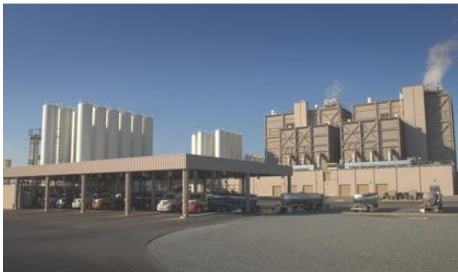
California Dairies, Inc.'s manufacturing facility in Visalia, CA
