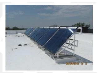
The **SunQuest 250**<sup>®</sup> utilizes evacuated tube technology. UV rays are absorbed by a proprietary coating on the inside collection tube, creating friction and heat that is then transferred by an internal heat pipe up and out through the unit header to interface with conventional hot water or space heating systems.
