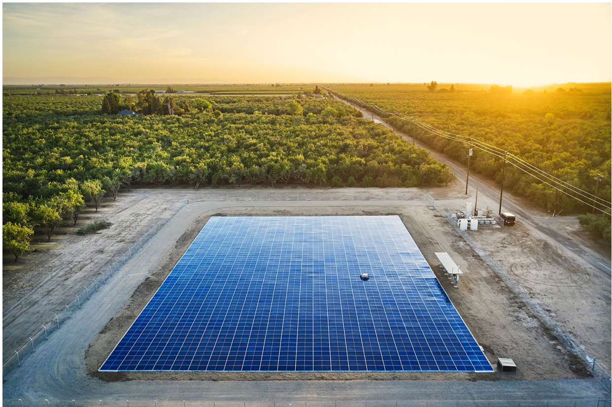
Figure 1 — Operating Erthos Plant in California
